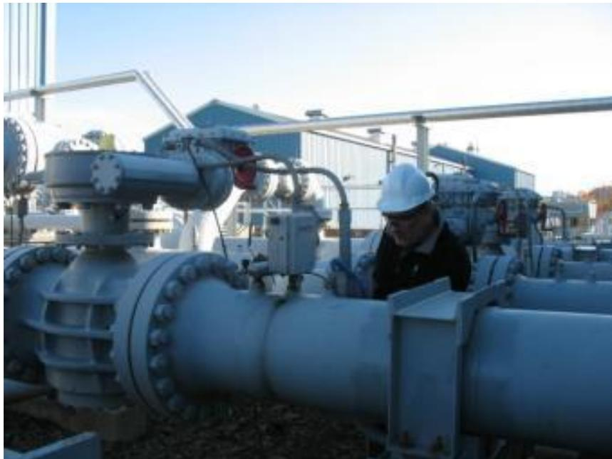
**Figure 6. Example unit isolation valve.**
