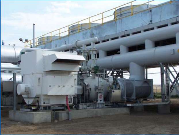
Turbine – Generator set & Air-cooled Condensers
