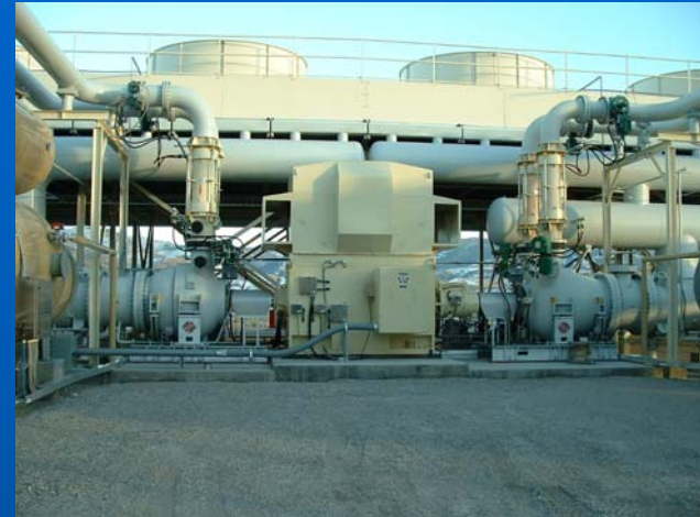
Turbine – Generator set & Air-cooled Condensers
