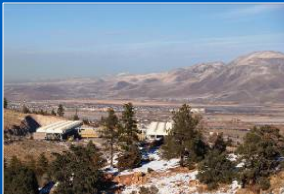
Geothermal Power Plants
