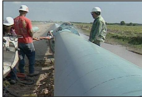
The natural gas industry uses several different types of pipe coatings. Historically, pipeline companies coated pipe with coal tar enamel or an enamel tape wrap. Today a fusion bond epoxy (FBE) coating is used most widely. FBE coating can be recognized by its light blue color, often seen on pipe being transported by rail or truck. Regardless of the type of coating used, the purpose is the same: prevent external corrosion by prohibiting moisture from coming into direct contact with the metal.
