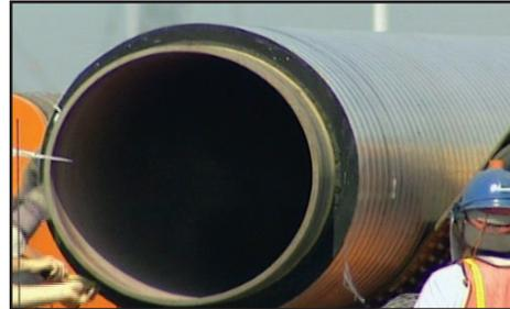
The thickness of the pipeline is determined by the maximum operating pressure (MAOP), and is based on published industry standards and federal regulations. The pipeline incorporates a design safety factor, prescribed by U.S. Department of Transportation (DOT) regulations, that is related to the type of construction and population density along the pipeline route.
