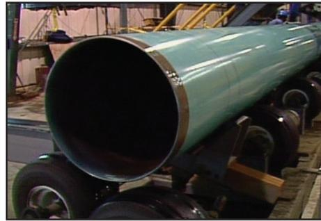
Prior to lowering the pipe into the trench, the coating of the entire pipeline is inspected to ensure it is free of defects.
