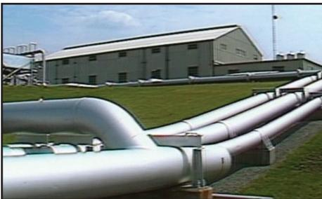
Some meter stations also regulate natural gas pressure and delivery volumes and are called meter and regulator stations (M&R). Pressure regulation equipment ensures that natural gas delivered into or out of a pipeline system is maintained within a specified pressure range. This is important for safety reasons, because transportation and distribution systems are designed to operate within specific pressure ranges.
