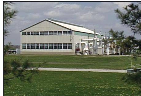
Pipeline companies install compressor stations along a pipeline route, typically every 40 to 100 miles. The size of the station and the number of compressors (pumps) varies, based on the diameter of the pipe and the volume of gas to be moved. Nevertheless, the basic components of a station are similar.
