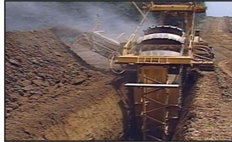
If the crew finds large quantities of solid rock during the trenching operation, it uses special equipment or explosives to remove the rock. The crew uses explosives carefully, in accordance with state and federal guidelines, to ensure a safe and controlled blast.
