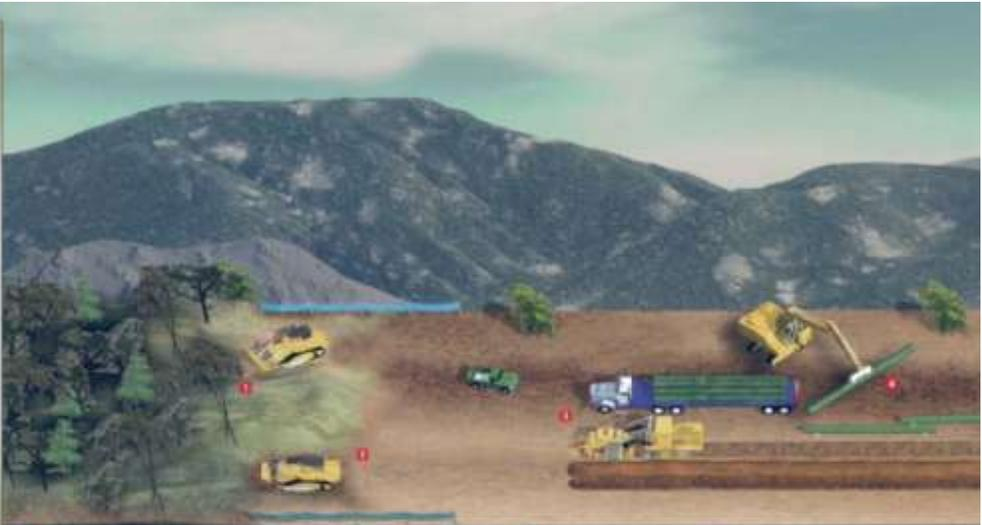
**1 Survey, setting out:** Marking the location of the pipeline ditch and the edges of the right-of-way.
