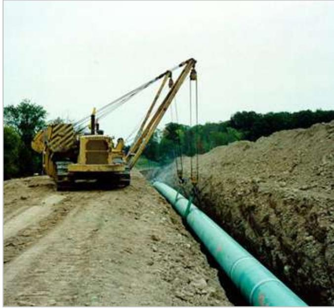
largest combined stresses that a pipeline will experience and use of appropriately deployed side booms ensures that the combined stresses remain below threshold levels established ASME.
