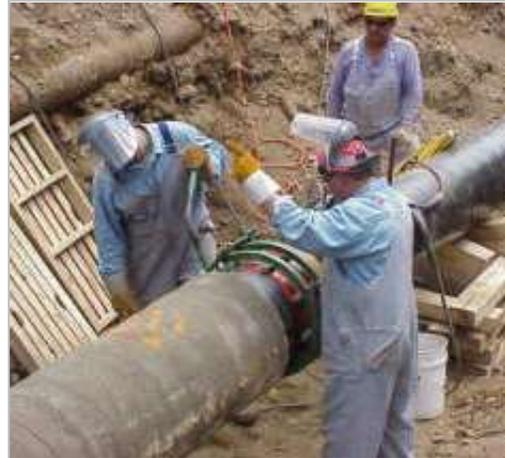
These obstructions and appurtenances, when in place, are quite rigid but must be connected with the remainder of the pipeline system. Typically, crews are dedicated to joining the appurtenances into the system by welding as well as applying coating at tie-ins.
