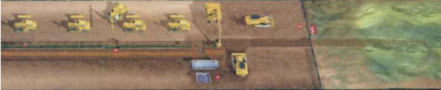
**9 Tie-in welding:** Individual pipe string with an end are joined to join the pipe strings with others) across obstacles across the pipe. HST inspection is performed after the pipe has been welded and the field data is recorded. Trench welding is also required at road crossings, flow crossings, and other intersections along the ROW where the main production welding pipe cannot access the joint.
