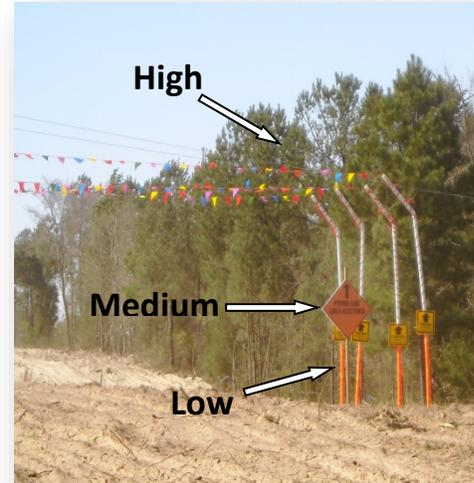
3. **Physical Barriers** – Non-conductive, highly visible devices (e.g., goal posts, barricade tape) set outside the limits of approach (limits will vary by jurisdiction, land restrictions and voltages) on both the coming in (upstream) and going away (downstream) sides.
